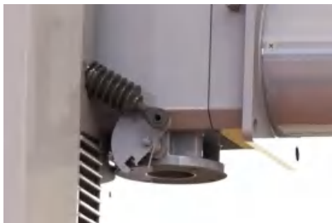
GDS 34-44Examples of Variable - Line Cam for Burners
