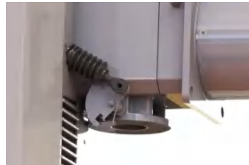
GDS/1 Example of Flange Connection for Burner Gas Valve Group
